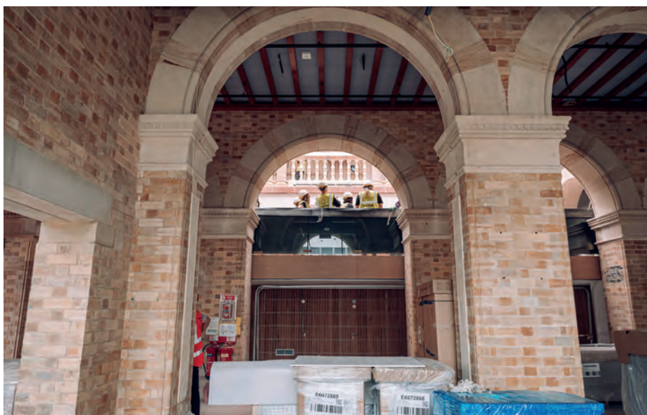
All change: The old Colston Hall has been undergoing renovation since 2011
